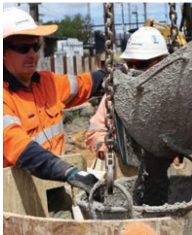
LEFT: Laing O’Rourke’s team working on the Level Crossing Removal Project.
