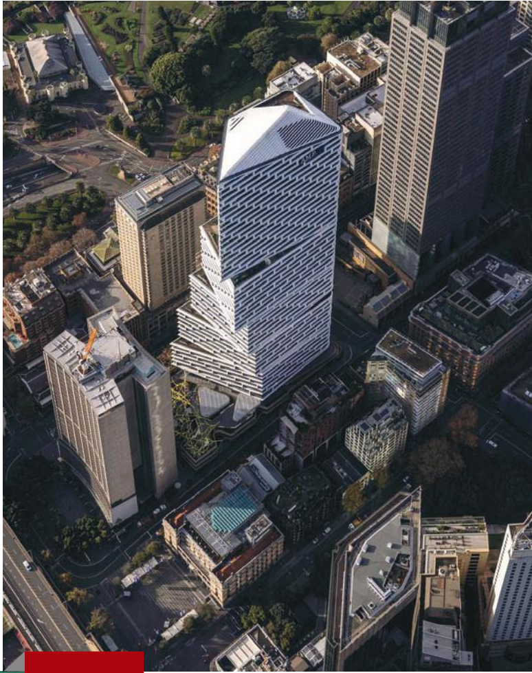
RIGHT: Quay Quarter Tower replaced the AMP Centre on Sydney Harbour.
