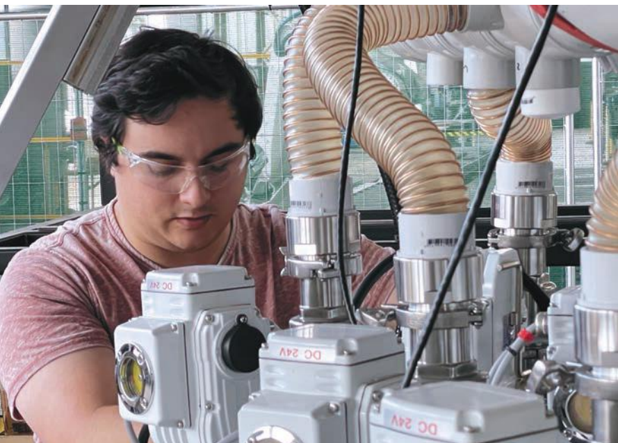
LEFT: Southern Green Gas's David Hedger adjusts a module.
