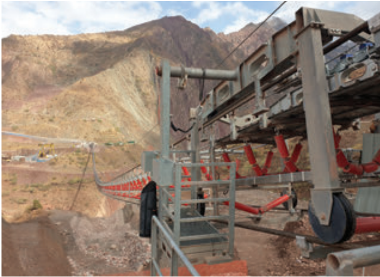
LEFT: The conveyor belt's support cables and slings prior to the belt itself being inserted.
