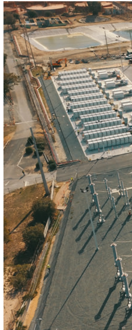
RIGHT: Kwinana Battery Energy Storage System 1 (KBESS1)
