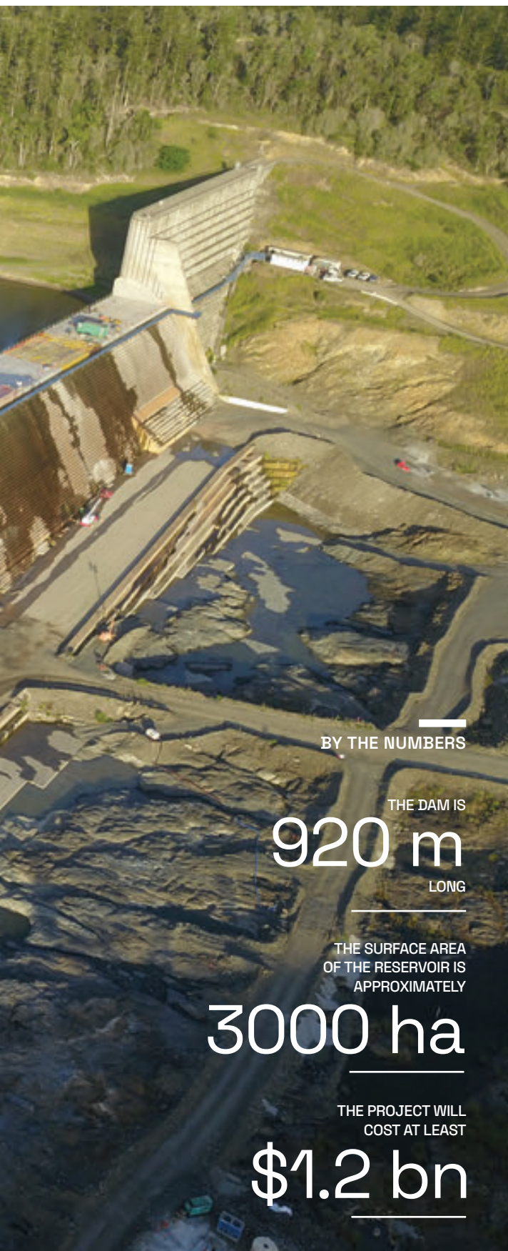
LEFT: Essential works were conducted in 2021 to ensure dam safety.
