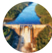
ABOVE: Paradise Dam Improvement Project concept design as of August 2024; Warragamba Dam. Images: Sunwater, Getty
