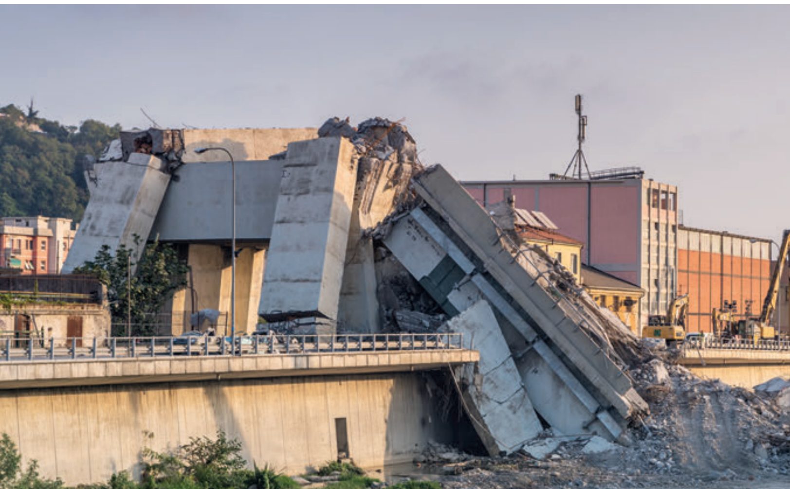
BELOW: What remains of collapsed Morandi Bridge connecting the A10 motorway in Genoa, Italy. The southern stays gave way explosively due to corrosion, with damage causing 43 casualties on 14 August 2018.
