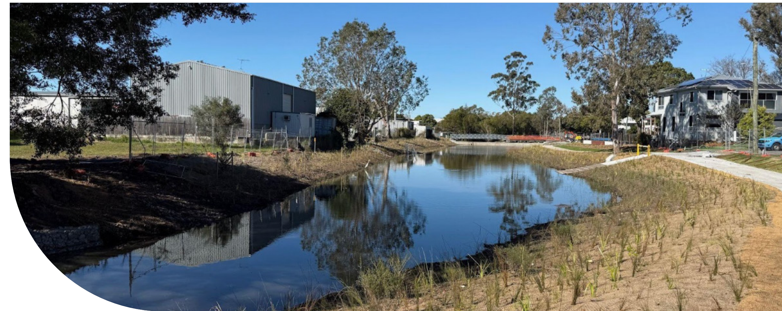
Above: Sediment Basin 1, post-planting works
