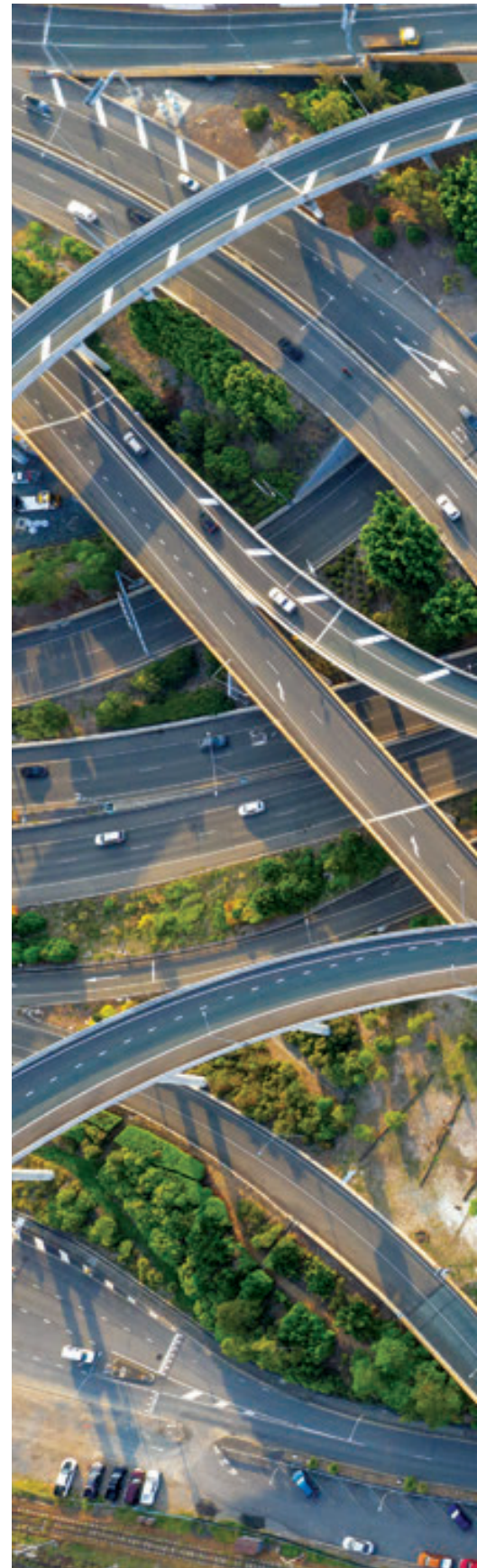
RIGHT: The Bowen Hills interchange in Brisbane plays a critical role in the city’s traffic network.
